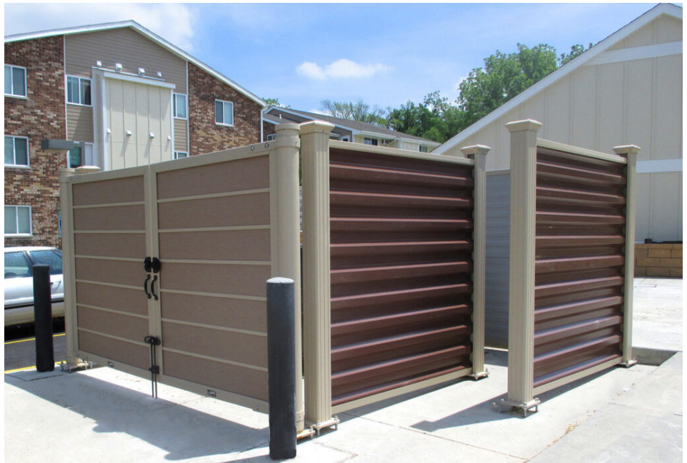
Waste Collection Facility Enclosure
