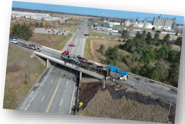
Figure 6: Investigations after the I-96 crash near M-52
